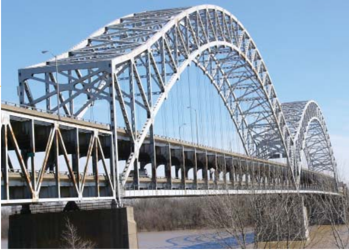
Sherman Minton Bridge, New Albany, Indiana
